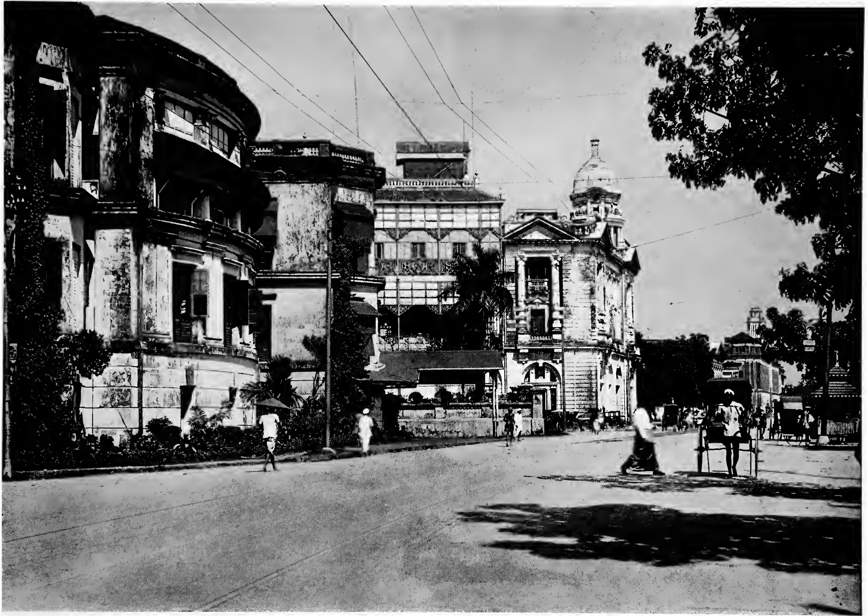
Strand Road, Rangoon.—Post Office, Imperial Bank of India. Custom House in distance
